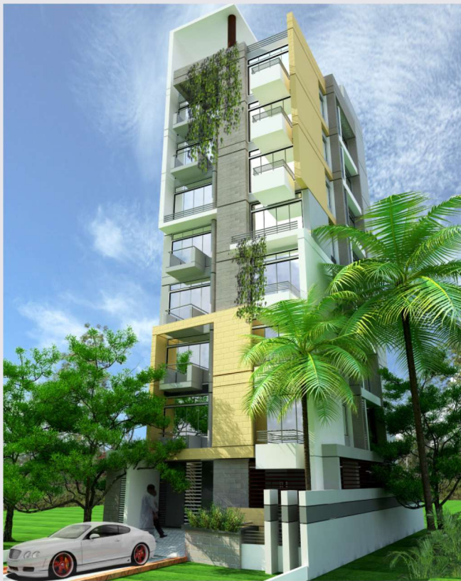
06 STORIED RESIDENTIAL BUILDING POLICE LINE NARAYANGANJ
